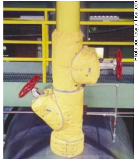
PHOTO A. A removable valve-insulation jacket.
