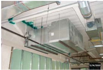
Photo is not of the actual damper but of a similar arrangement but with an electric actuator
