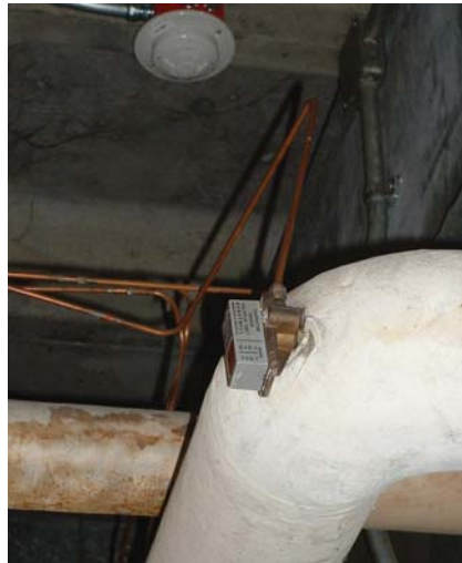
PHOTOS A1 and A2. One-pipe pneumatic technology encountered on a recent retrocommissioning project. The one-pipe pneumatic transmitter (left) and receiver controller (right) serve the central systems in a lab building on a large college campus.
