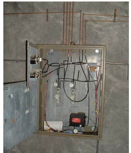
PHOTOS A1 and A2. One-pipe pneumatic technology encountered on a recent retrocommissioning project. The one-pipe pneumatic transmitter (left) and receiver controller (right) serve the central systems in a lab building on a large college campus.
