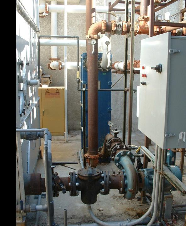
The Heat Exchanger and Boiler
